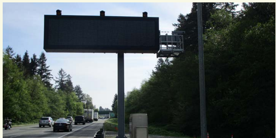
This Variable Message Sign on northbound I-5 approaching Mounts Road near DuPont is part of the larger I-5/Joint Base Lewis-McChord (JBLM) Corridor Improvements project and will improve future corridor congestion management and safety in the area.
